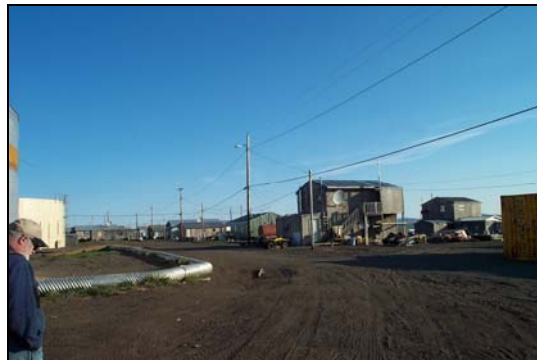
Typical structures in Kivalina
