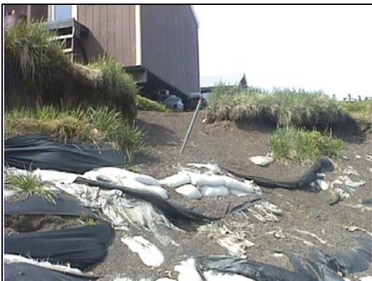
Undermined building on Kivalina
